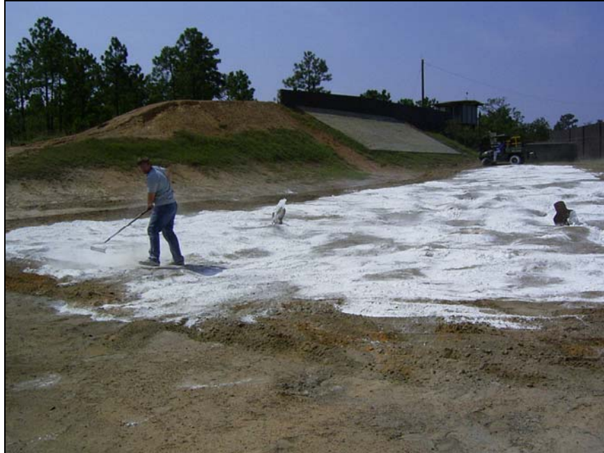
Figure 6. Applying \text{Ca}(\text{OH})_2 by hand
