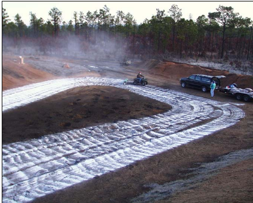
Figure 7. Applying \text{Ca}(\text{OH})_2 with a drop spreader
