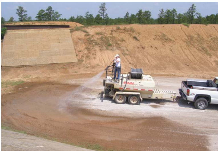
Figure 18. A hydro seeder was used after the final lime application to evaluate its effectiveness for dust control
