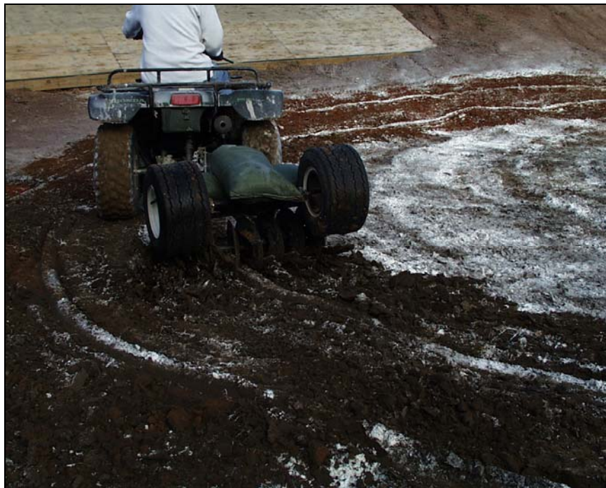
Figure 9. Using a disc to mix the lime into the Fort Jackson HGR soil to a depth of approximately 6 in
