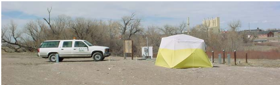
Figure 9. Final Grade Showing Sampling Shelter and Rectifier.
