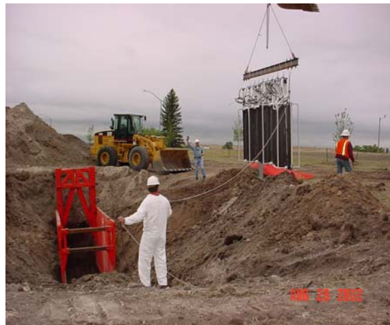
Figure 7. Placement of Nine Linked E-Barrier Panels into the Trench.
