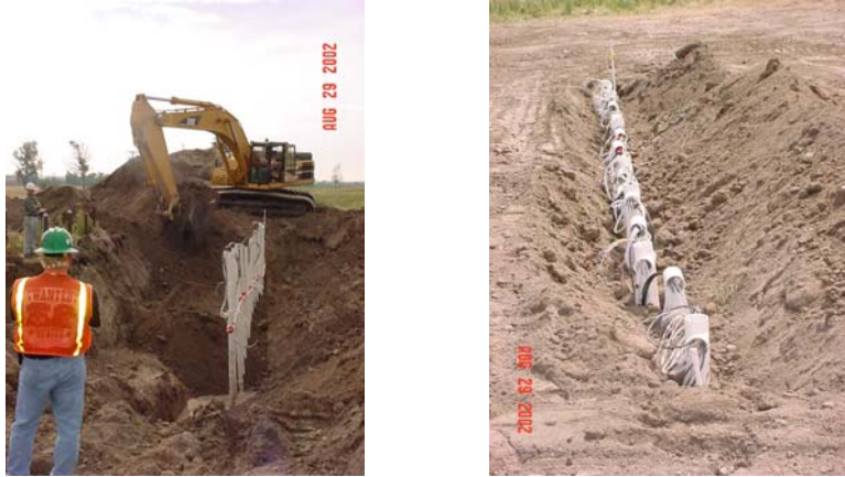
Figure 8. Backfill and Shallow Completion.
